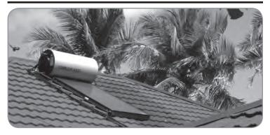
Active solar systems use special solar collectors that look like boxes covered with glass. Dark-colored metal plates inside the boxes absorb the sunlight and change it into heat. (Black absorbs more sunlight than any other color.) Air or a liquid flows through the collectors and is warmed by this heat. The warmed air or liquid is then distributed to the rest of the house just as it would be with an ordinary furnace system.
